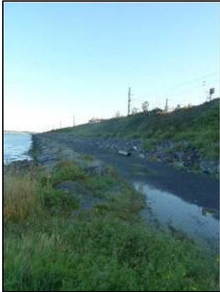
Text Figure 4.24. Existing Stoned Access Track to South of Viaduct.
