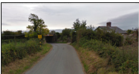
Text Figure 9.7. Railway Underpass on Corballis Cottages Road.
