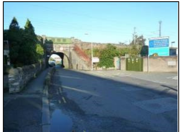
Text Figure 4.21. Bissets Railway Bridge.
