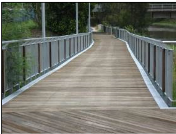
Text Figure 2.3. Timber Boardwalk Surface Finish.
