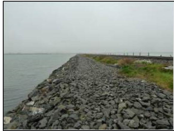
Text Figure 4.25. Stoned Area to North of Viaduct.
