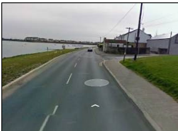
Text Figure 4.12. Junction of Texas Lane and Bissets Strand.
