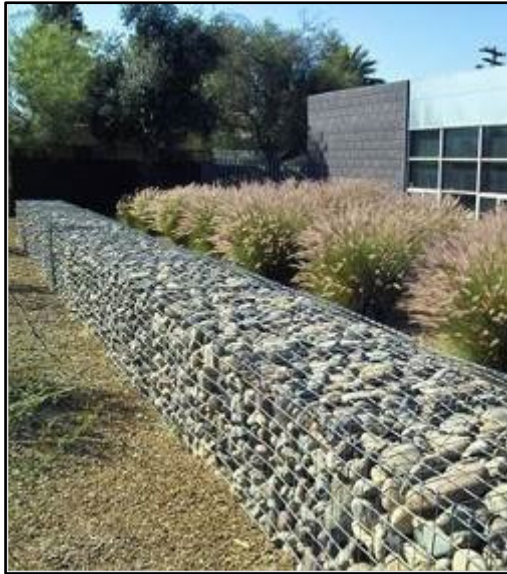
Text Figure 2.8. Gabion Wall Example.
