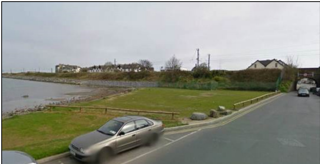
Text Figure 4.23. Photograph of Green Area at Bissets Strand Prior to Construction of Irish Rail Site Compound.
